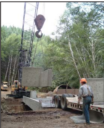
Installation of the W. Fork Millcoma Bridge, Elliott State Forest
