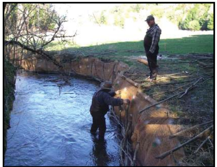
Fishermen Bob Miller and Jacob Praus working on willow wall project on Daniels Creek, January-February, 2008
