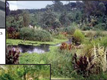
Constructed wetland to treat pollutants in stormwater runoff
