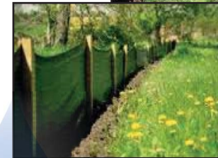
Sediment fence to prevent erosion from impacting near-by waterways
