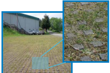
Paving bricks at Millicoma Middle School, Coos Bay, Oregon.
