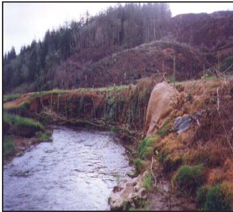
Willow wall construction helped to shade the stream and lower the water temperature. (Photo taken in 1997.)
