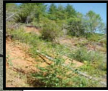
Landslide that occurred in the Upper Wood Treatment reach during winter 2006 / 2007.
