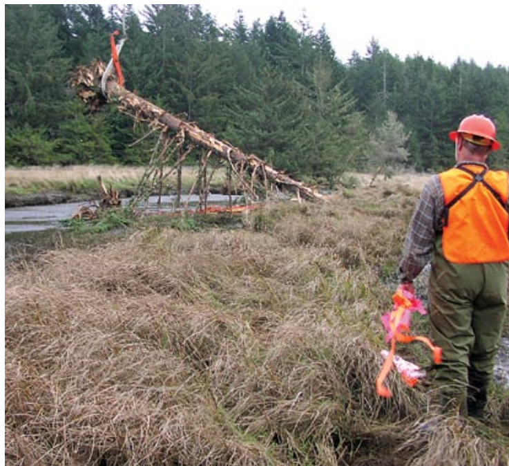
Top right: The helicopter lifts the trees in their entirety to the stream for placement. Placement of whole trees in-stream is more cost-efficient and provides more complexity in the fish habitat.
