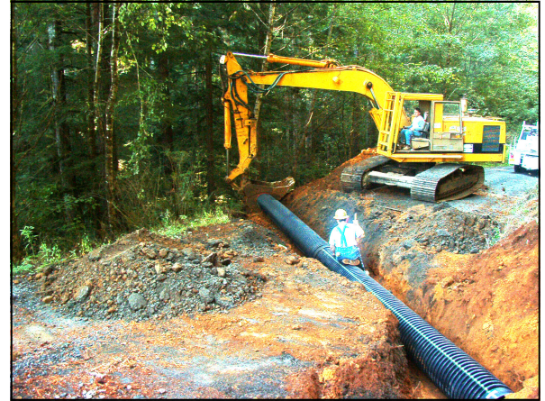
Installing ditch relief culvert on county road near Daniel's Creek.
